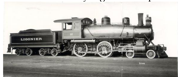
Engine #17 4-4-0 purchased new from Baldwin
